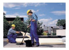
✓ Flat roof insulation panels: can be walked upon and are easy to lay.
