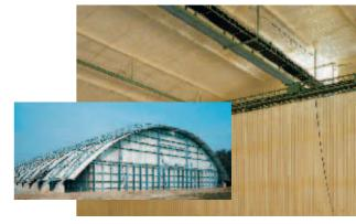
△▷ Warehouse in northern Germany: inside insulation with thin layers of material for a big increase in thermal insulation.
