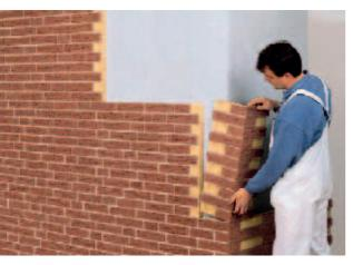
⊂ Clinker insulation panels made of Elastopor H are used to refurbish houses: heat loss is reduced and the façade is improved at the same time. A further benefit: the external dimensions of the building only increase marginally.
