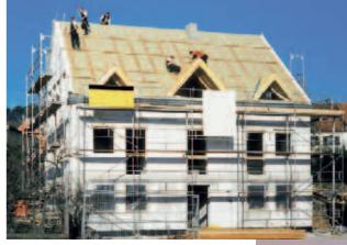
$\triangle$  Spray foam for roofs is the ideal solution for difficult geometric shapes: Elastopor H coating is free of thermal bridges and can be walked upon.
