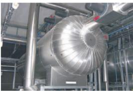
$\Delta \nabla$  Lined "in situ" with Elastopor H spray foam: the double-wall reactor including the necessary piping.
