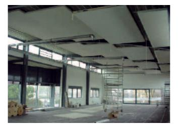
Elastopor H combined with Micronal PCM® (phase change material) SmartBoard® creates new potential areas of application eg as construction material for "energy costfree air conditioning systems": wax, micro-encapsulated as minute beads and embedded in wall boards provides additional cooling capacity in the event of increased heat. Thus it forms the basis for regenerative and low-cost cooling concepts such as cooling with ground water.
