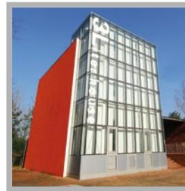
■ The Korean Three Liter House with insulation panels made of Neopor® and gypsum plaster containing Micronal®
