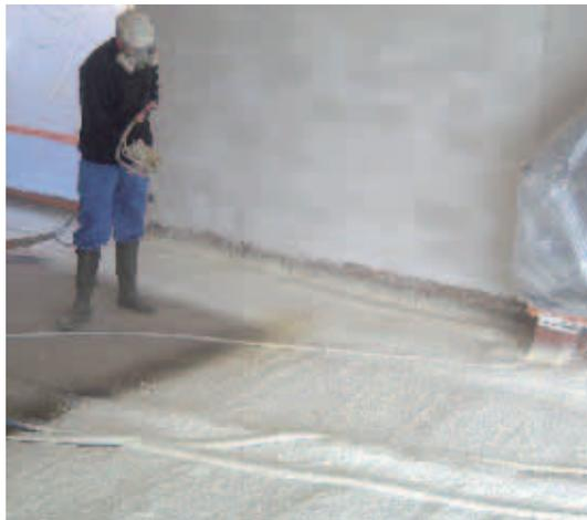
▷ Floor insulation with spray foam: rational processing without thermal bridges.
