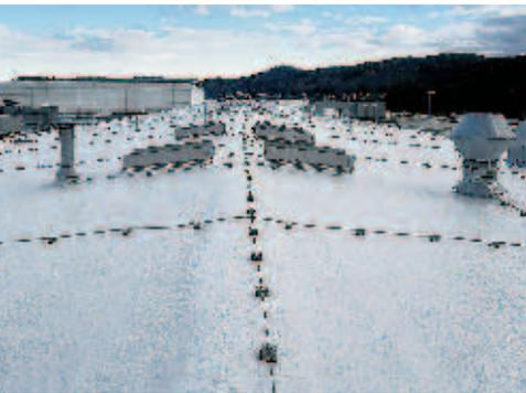
△ Spray foam for roofs is the ideal solution for difficult geometric shapes: Elastopor H coating is free of thermal bridges and can be walked upon.
