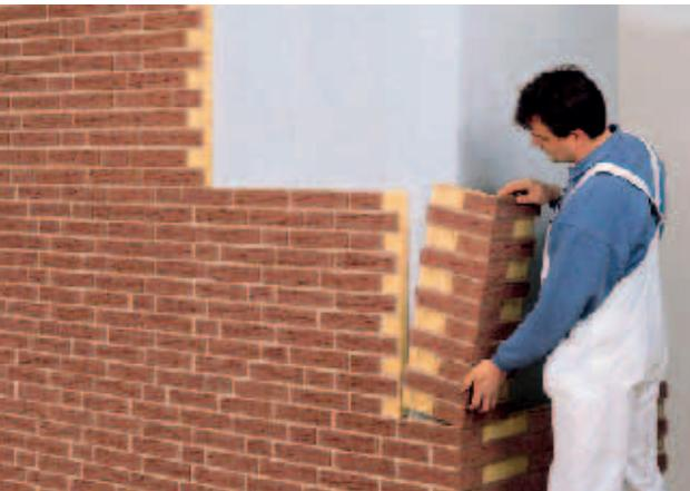
◁ Clinker insulation panels made of Elastopor H are used to refurbish houses: heat loss is reduced and the façade is improved at the same time. A further benefit: the external dimensions of the building only increase marginally.
