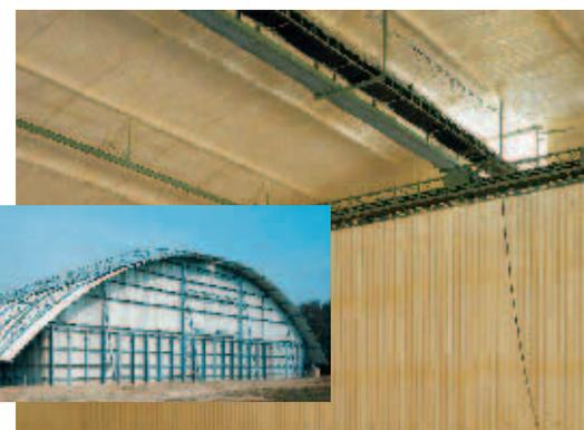
*△▷ Warehouse in northern Germany: inside insulation with thin layers of material for a big increase in thermal insulation.*
