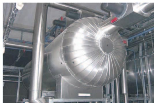
*△▽ Lined "in situ" with Elastopor H spray foam: the double-wall reactor including the necessary piping.*
