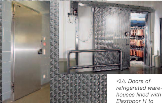
◁△ Doors of refrigerated warehouses lined with Elastopor H to prevent heat loss.
