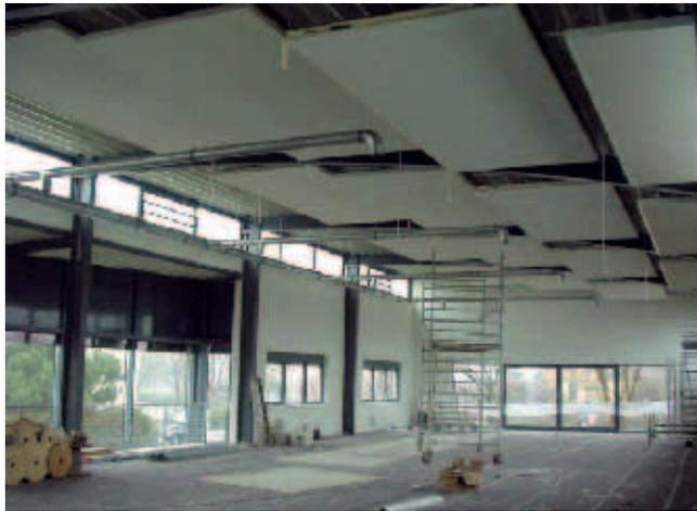
**Elastopor H combined with Micronal PCM® (phase change material) SmartBoard® creates new potential areas of application eg as construction material for "energy cost-free air conditioning systems": wax, micro-encapsulated as minute beads and embedded in wall boards provides additional cooling capacity in the event of increased heat. Thus it forms the basis for regenerative and low-cost cooling con-**
