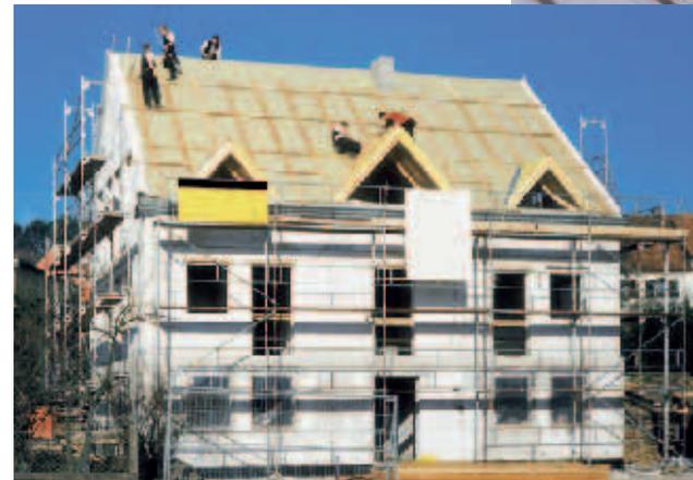
△▷ Steep roof insulation panels made of Elastopor H/Elastopir on, under or between the rafters for insulation without thermal bridges. Easy to process.
