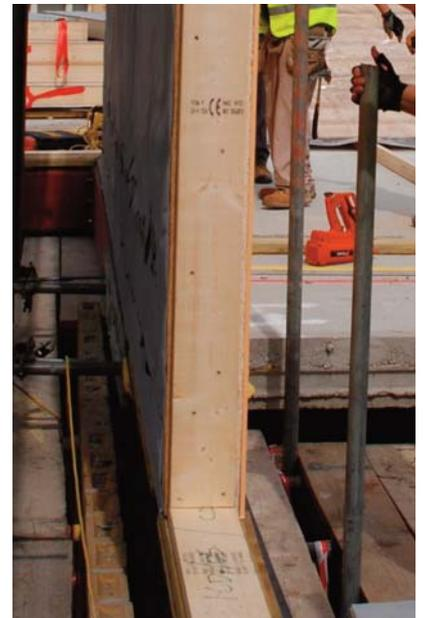
Racking resistance of a SIP wall is typically 50% greater than that of a timber studwork wall sheathed with one layer of 9mm OSB. Therefore a low rise building designed to be constructed with loadbearing timber studwork, should also work as a loadbearing SIP structure. A structural engineer would need to confirm this by calculation.
