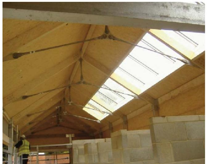
Coverings for pitched SIP roofs can be any type of covering that may be used on any other type of roof (e.g. tiles, slates, profiled metal etc). A ventilation void must be provided between the SIP and the roof covering, so the use of counter battens before tiling battens, profiled metal roofing or any other covering should be considered. Roofing battens should be fixed to the SIP roof with the use of screws.
