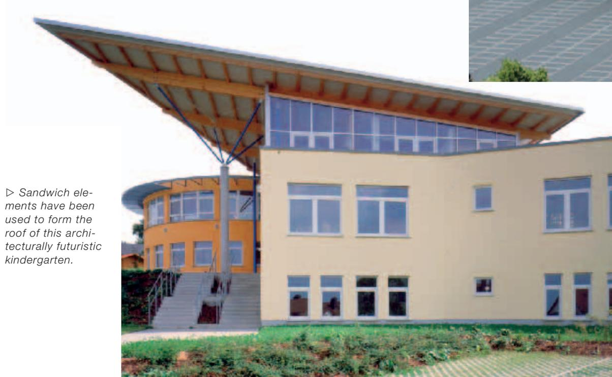
◁ The design of this innovative multi-purpose building was possible with sandwich elements.
