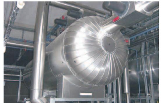
△▽ Lined "in situ" with Elastopor H spray foam: the double-wall reactor including the necessary piping.
